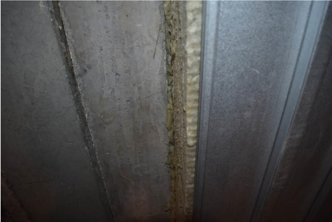
Photo No. 7 The test specimen seen from unexposed side at fixed edge
