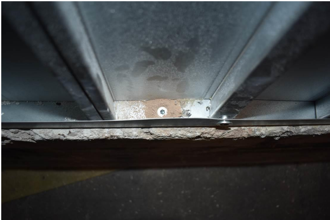
Photo No. 4 The test specimen seen from exposed side at lower edge – attached to the concrete frame with screws
