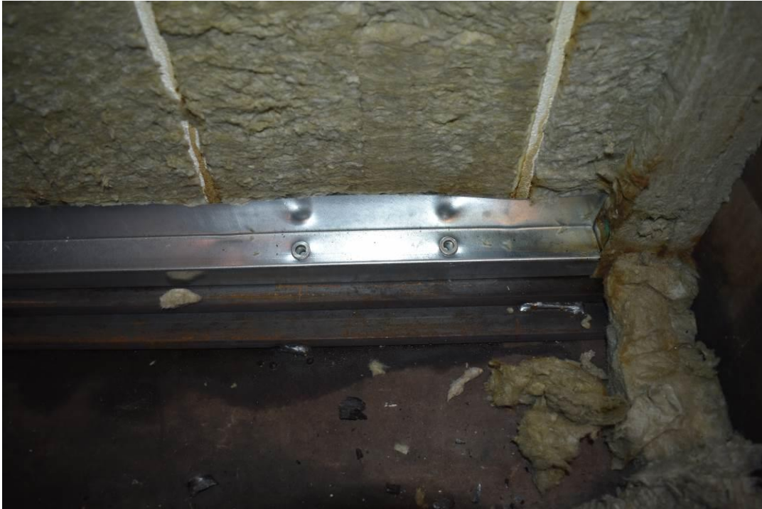
Photo No. 13 The test specimen simple supported in the test frame after testing
