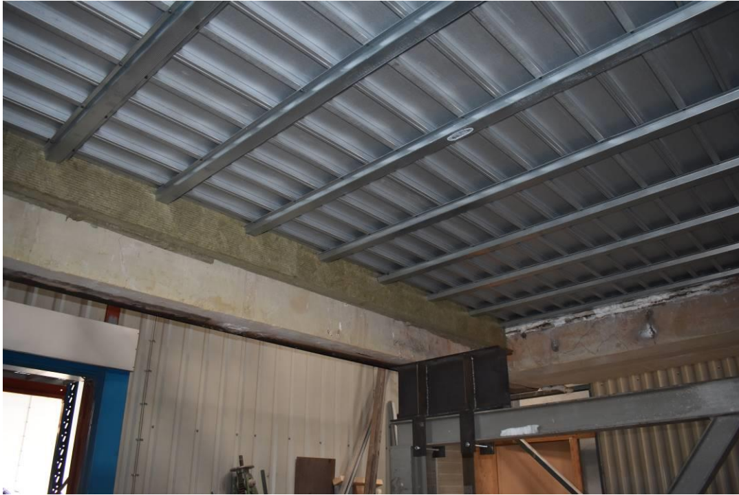
Photo No. 7 Mounting of hat profiles with cc 400 mm on exposed side of the test specimen
