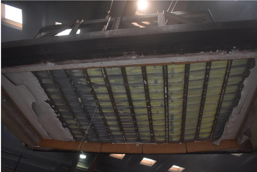
Photo No. 19 The test specimen seen from exposed side after testing
