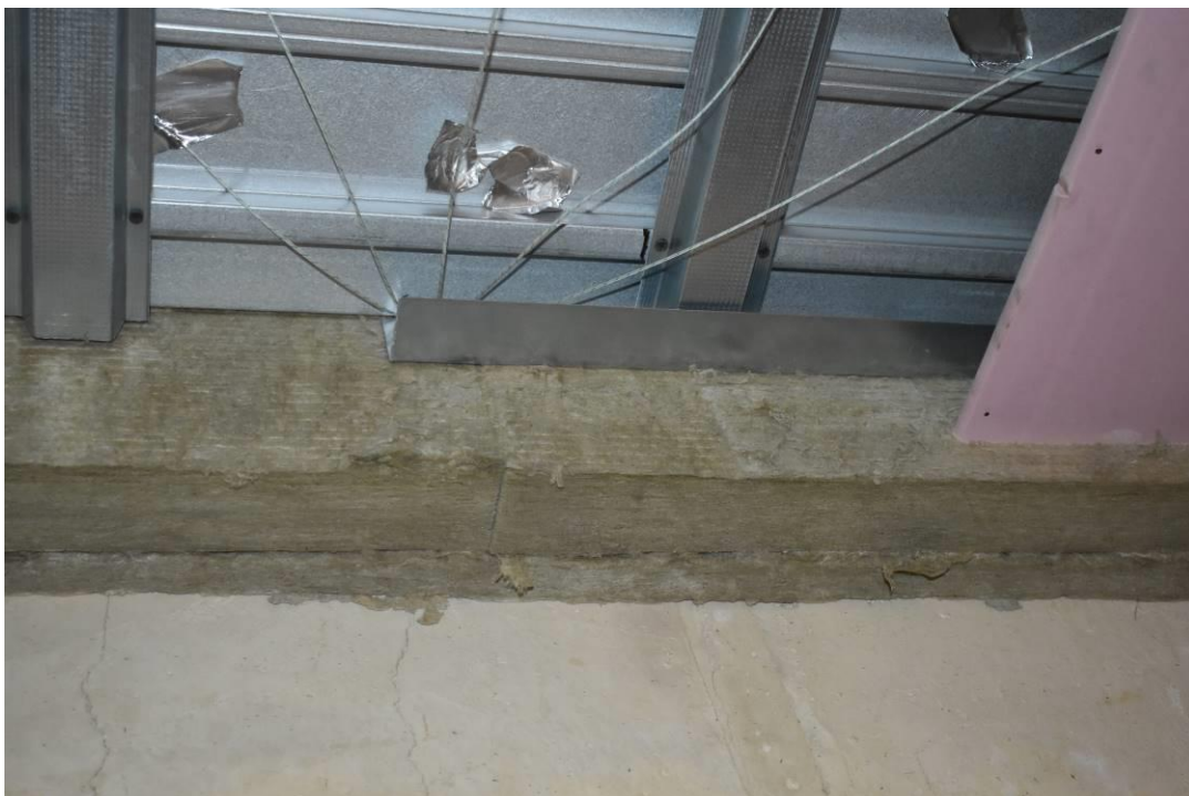
Photo No. 10 A 50 x 50 mm steel profile was mounted on each side of the test specimen as support for the gypsum plaster boards
