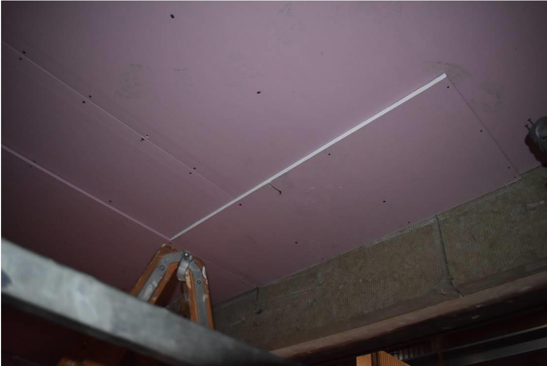
Photo No. 13 Mounting of second layer of gypsum plaster boards
